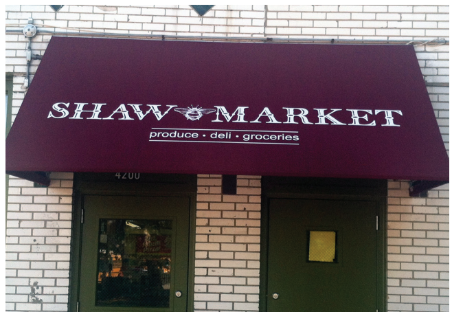
Close-up of improved store awning.
