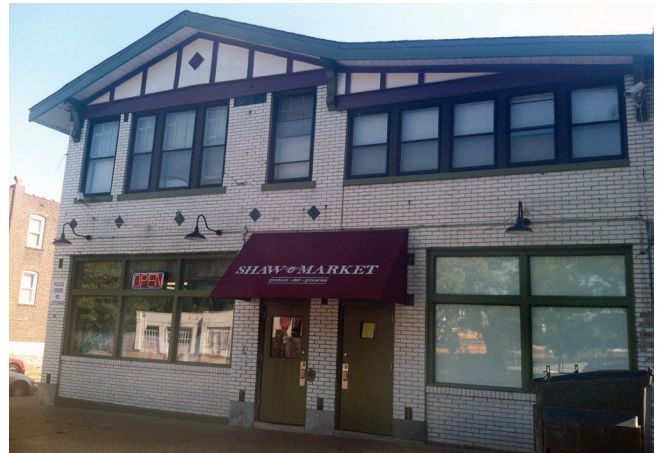
After storefront improvements.
