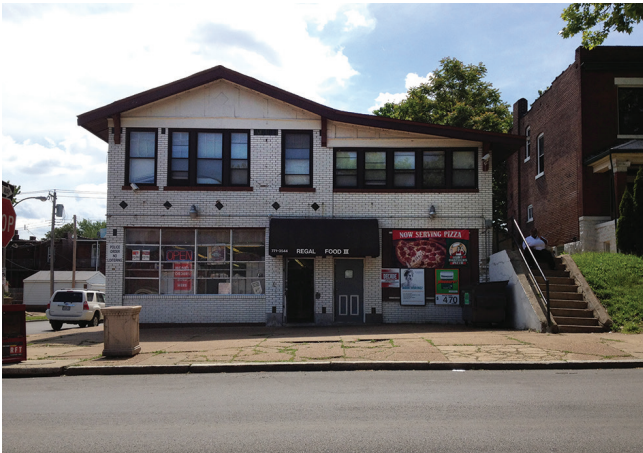
Before storefront improvements.
