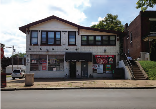
Before storefront improvements.
