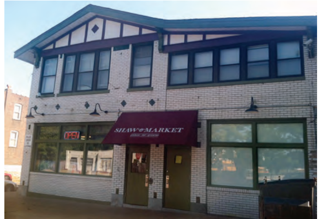
After storefront improvements.
