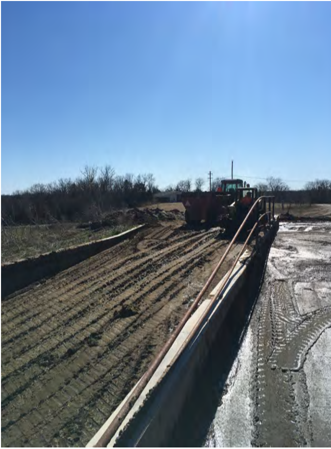
Figure 7b. PPSB ramp and adjoining sand lane.
