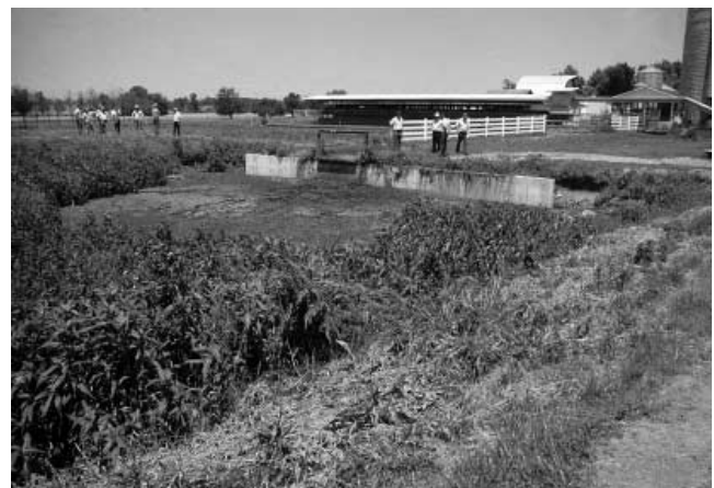
Figure 3. Without agitation a pit can become overgrown.
