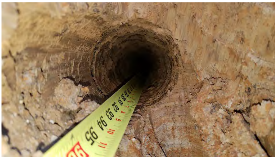
Figure 2. Mole channel 20 inches below the soil surface with a 4-inch diameter in a claypan soil.
